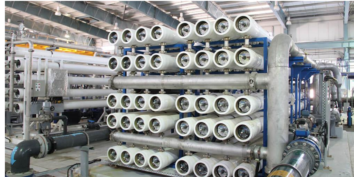
Reverse osmosis plant to enable full water recycling on site
