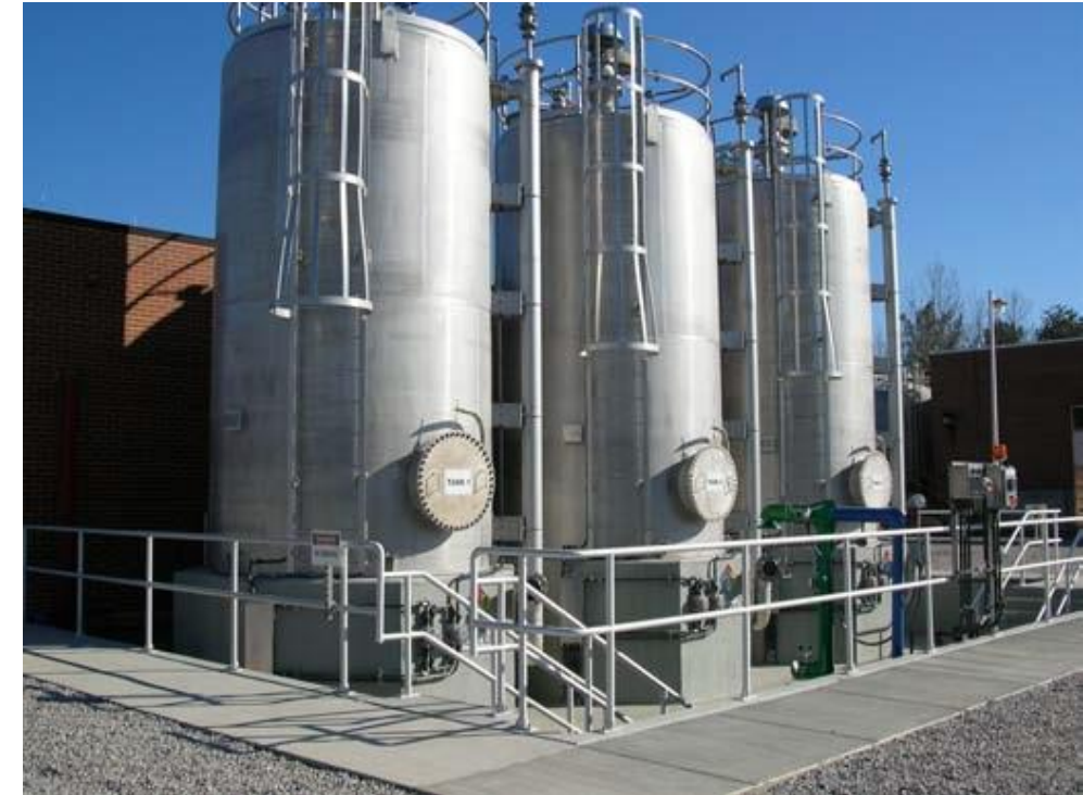
Example methanol storage tank infrastructure to be used at the site
